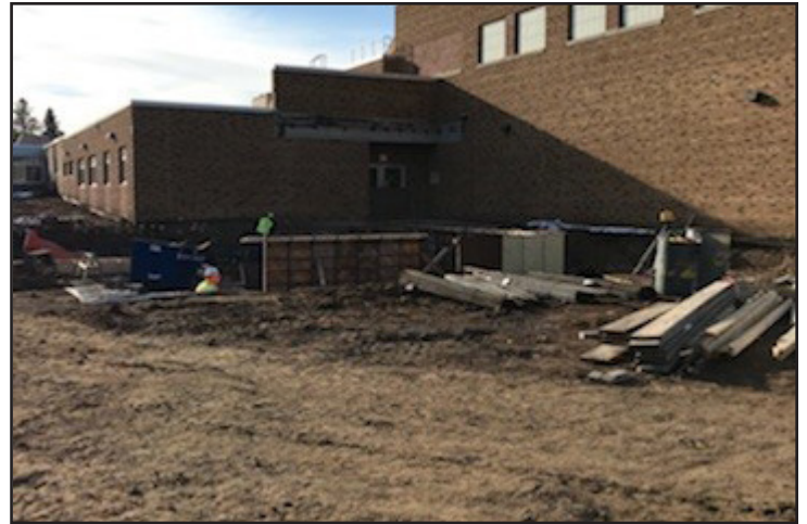
Upper left: Forming foundation walls
